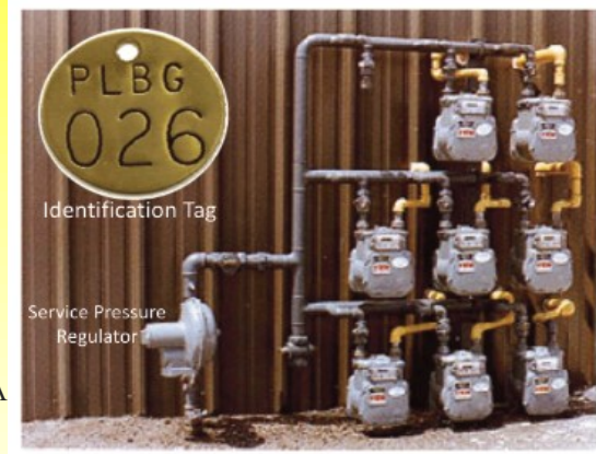
FIGURE 1208.7.4 MULTIPLE METER INSTALLATION AND METER TAG
